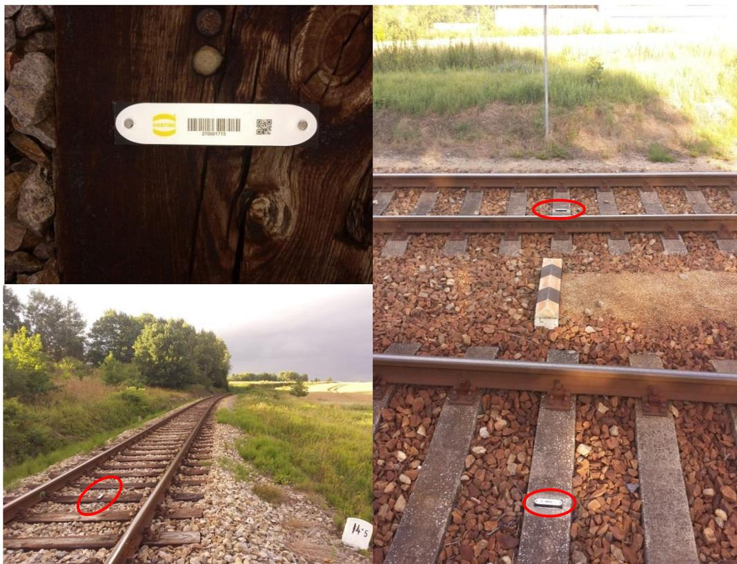
**Figure 4: RF ID tags as installed in the track**
